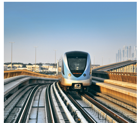
Metro/Train Road Tunnels
